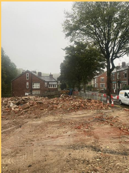
Removal of the waste following completion of the demolition work
