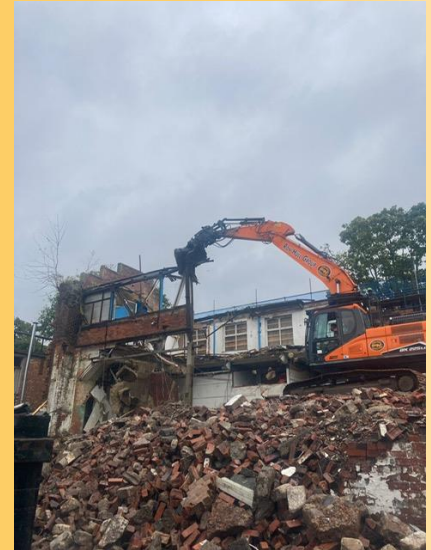
Demolition by 25t machine
