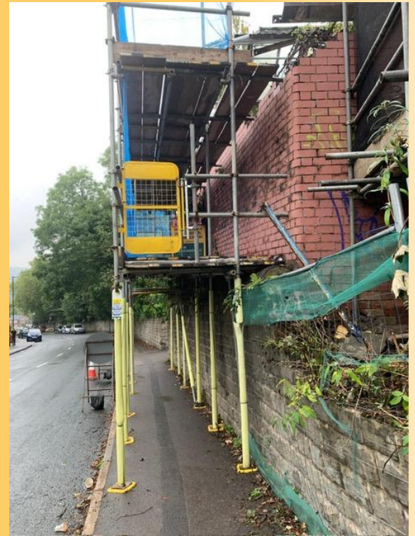
Pedestrian walk through scaffold at the Derbyshire Lane elevation
