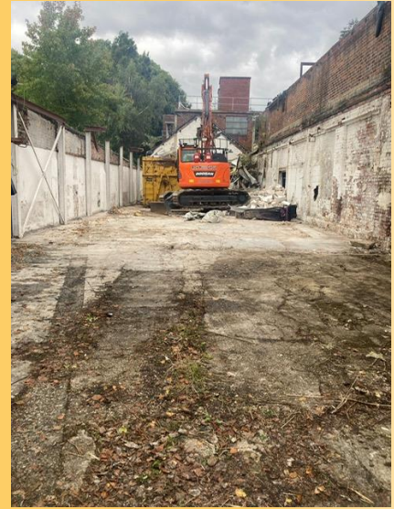
Demolition by 14t machine
